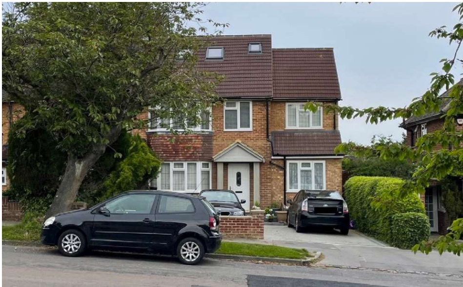
Figure 1: photograph of the front of property from The Ruffetts (note this image was taken more recently than Figure 2 below)
